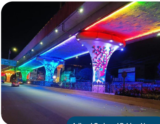
Adivasi Godavari Bridge, Nagpur
